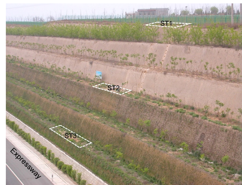
(a) Site photograph showing the monitoring locations on the slope
